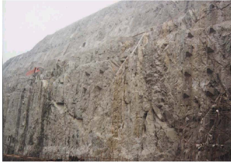
Fig. 11. A reinforced wedge in the ship lock (Three Gorges Project).
